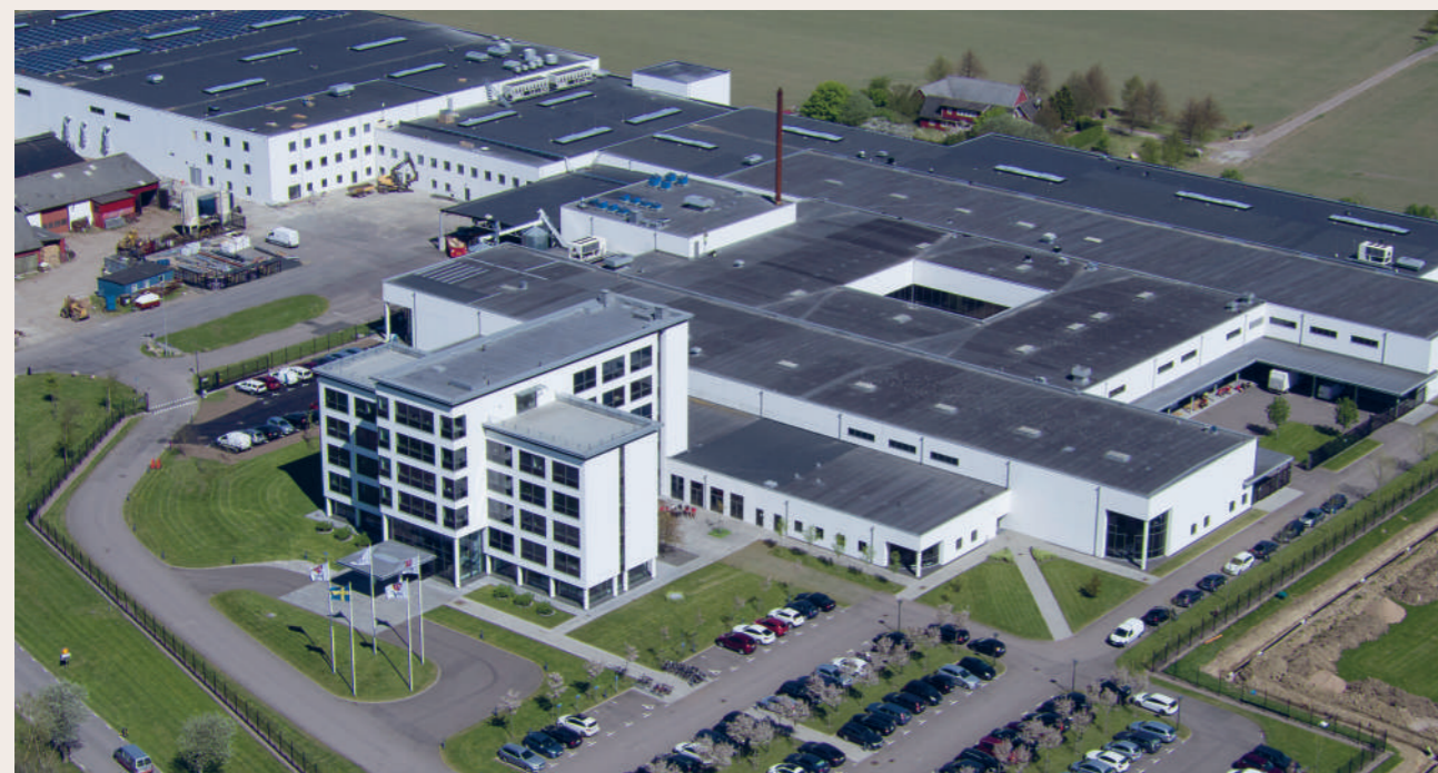
Our parent company Välinge Innovation owns and manages a modern, state-of-the-art production facility in Viken, Sweden
